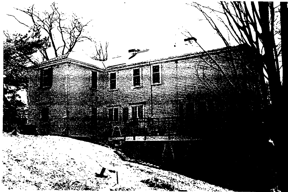
REAR / NORTH SIDE
