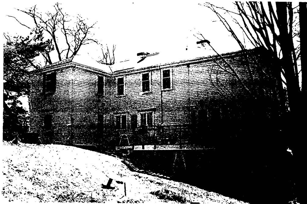
REAR / NORTH SIDE
