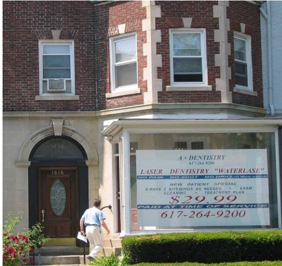
Beacon Street, Brookline Window coverage exceeding 30%
