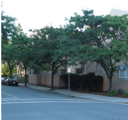
Centre Street, Brookline Example of 6' high fence in an M District
