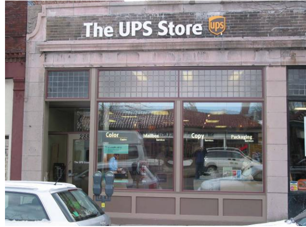
Brookline Village Storefront w/ more than 75% glazing
