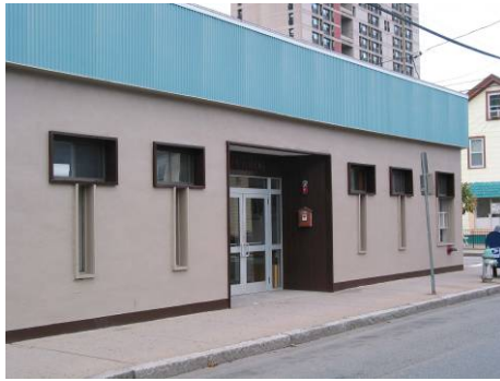
Cambridge, MA Storefront w/ less than 75% glazing
