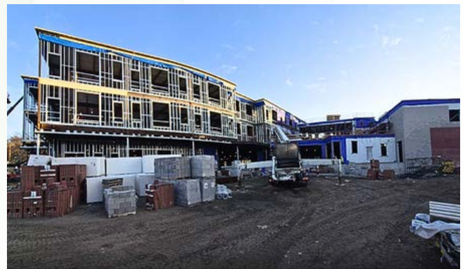
Countryside Elementary New Construction
