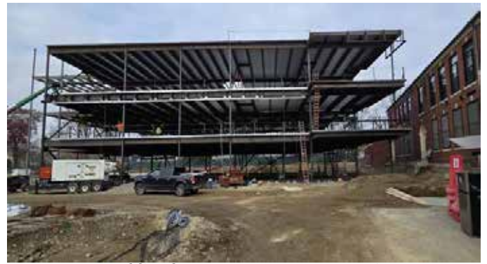
Franklin Elementary New Construction
