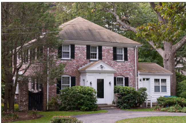
Although constructed with different materials, the wood-framed addition located in Auburndale complements and “defers” to the original brick house. The addition has a similar roof form and multi-light windows to the main house and the wood siding complements the projecting central entrance.
