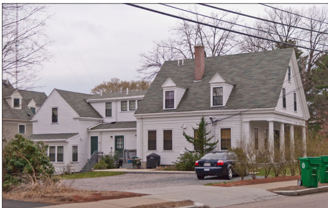
The series of additions at this home in Newton Upper Falls shows the expansion of the original house over time. The additions share similar forms and materials to the historic house, simplified detailing, and are largely concealed behind its main block.
