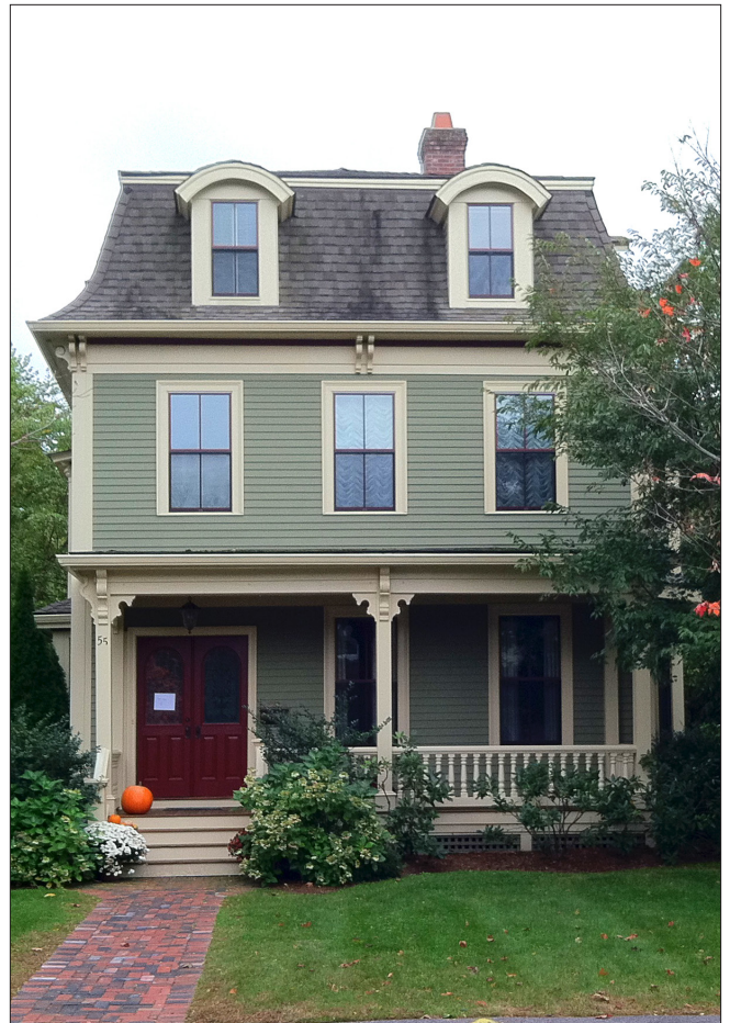
This vernacular Second-Empire home has a mansard roof with arch-headed dormers. The projecting roof cornice features paired brackets similar to those found at the porch posts.
