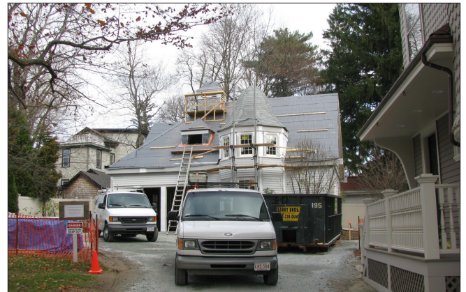
The work at this carriage house, at 43 Fairmount Avenue, is being funded in part through state and federal tax credits.
