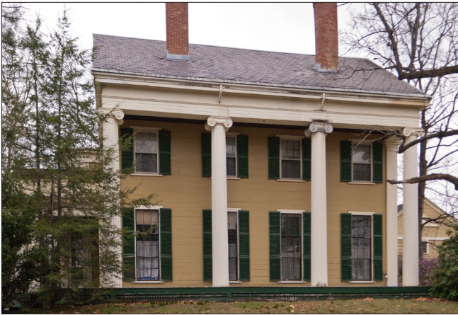
The Greek Revival style, which typically includes large porticos and classical columns as in this Local Landmark at 35 Webster Street, was popular in the first half of the 19th century.
