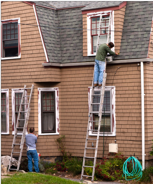
General maintenance, including repainting of woodwork, is essential for preserving original building fabric and unique architectural elements and details.
