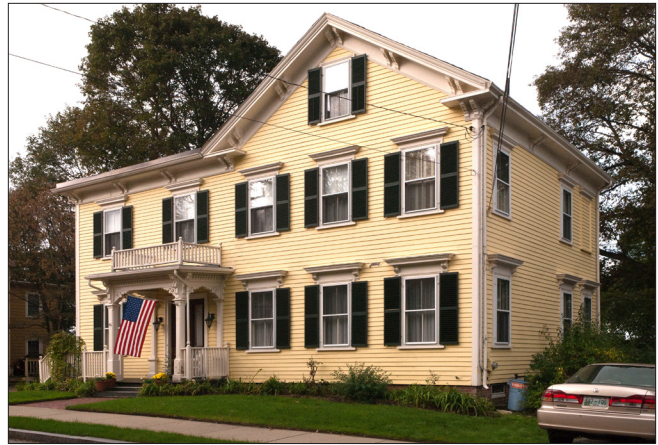
Newton's homes, such as this one in Upper Falls, often have exterior details such as cornices, porches and window surrounds. Regular maintenance and repainting can prolong the life of historic materials.
