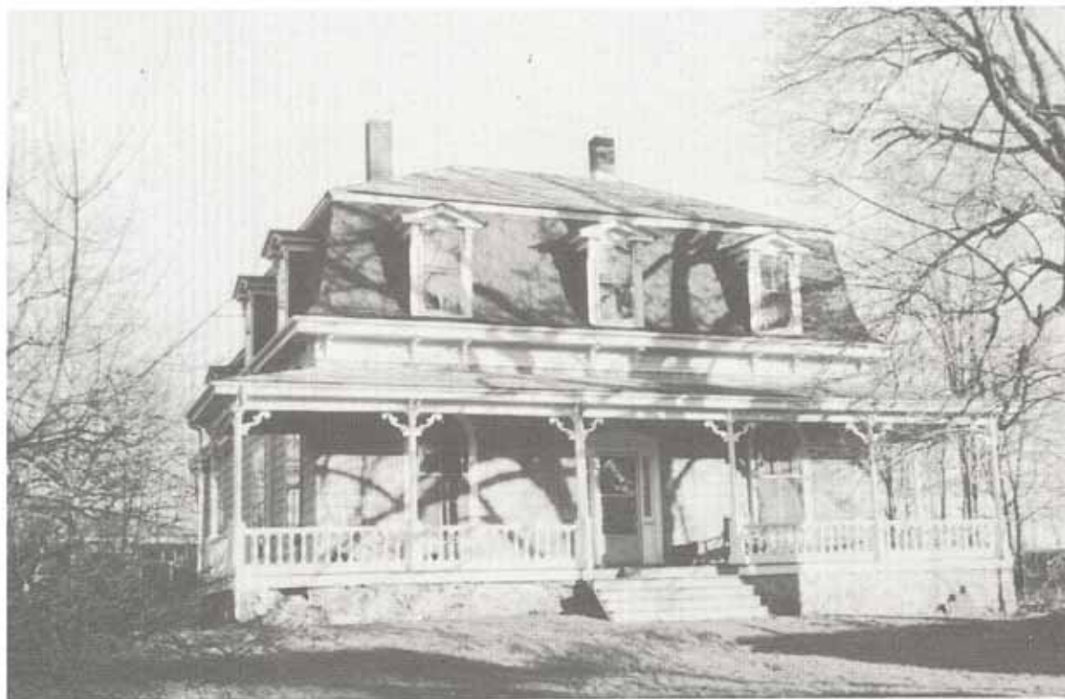
Figure 17. Newton Highlands: 450 Winchester Street, c. 1865
