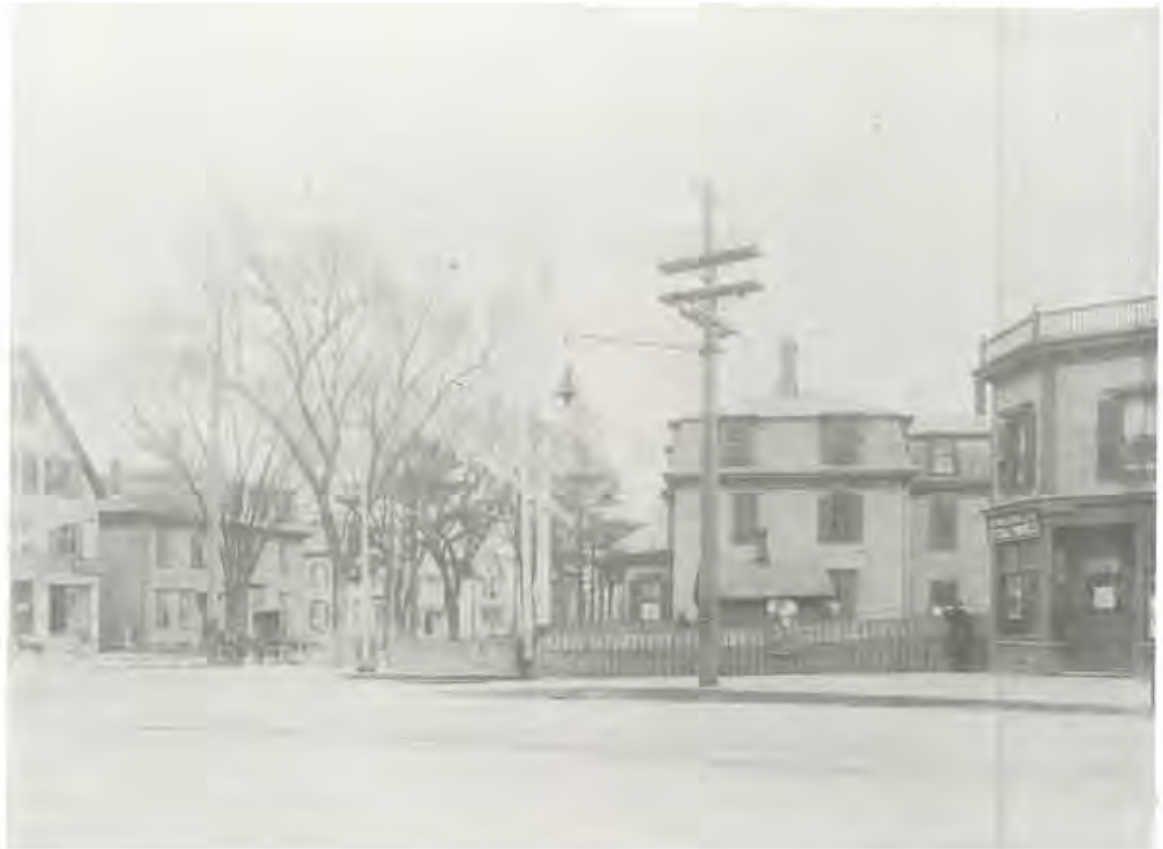
Corner of Lincoln and Walnut Streets, looking south, 1902
