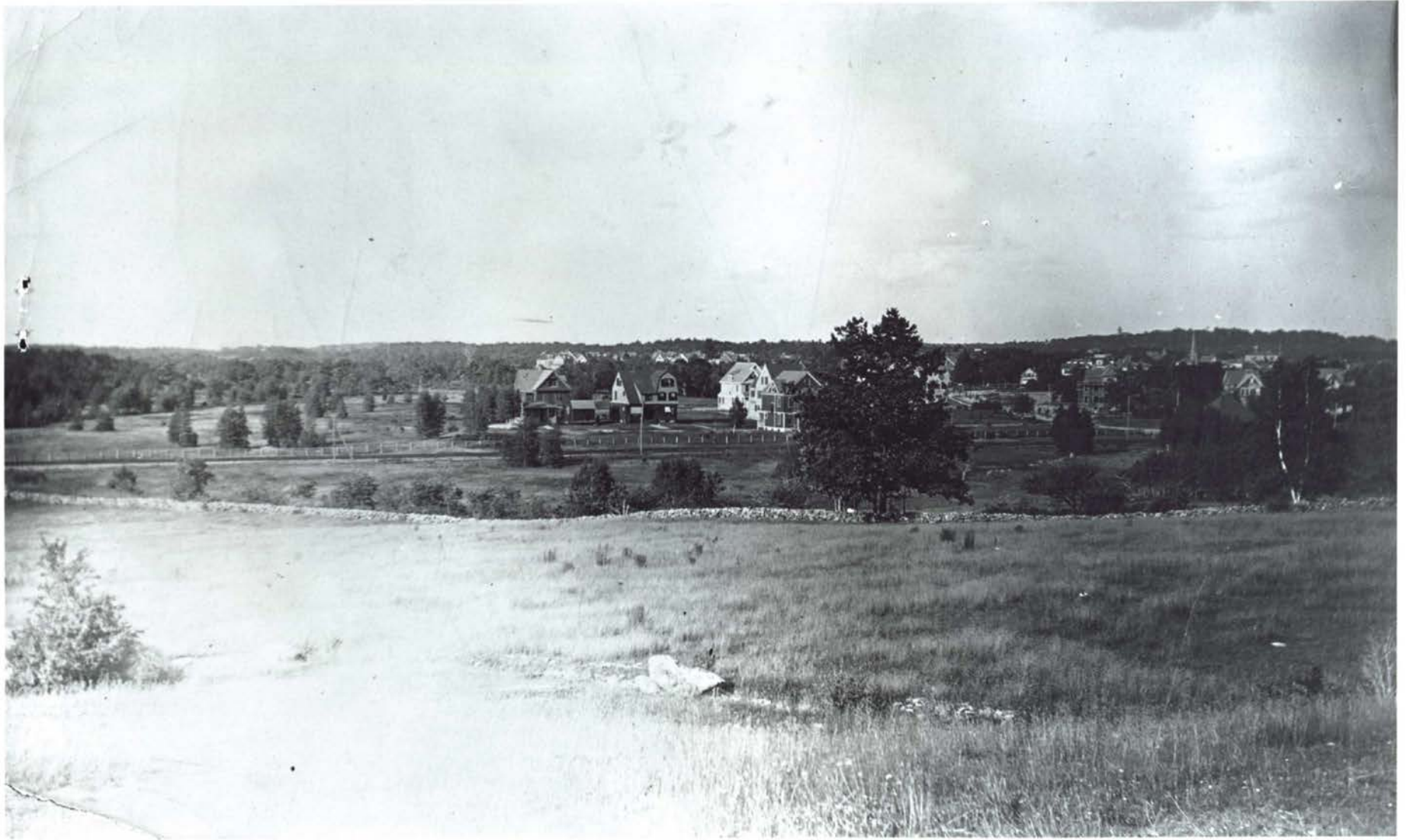
Newton Highlands, near Eliot station, 1890's
