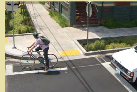
Stormwater management in curb extensions. Source: Sustainable City Network
