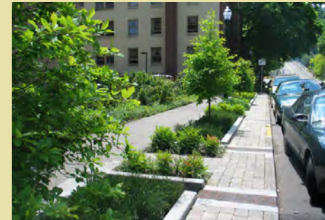
Sidewalk stormwater infiltration facility in Portland. Source: Green Infrastructure Digest
