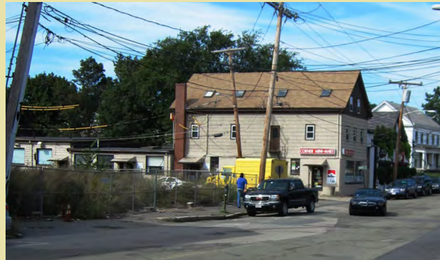
Fig. 10-14. View of Border Street from Elm Street
